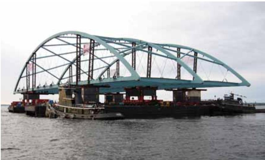
On August 27th of 2006 the PUMA and the RESOLUTE, along with tugs and barges from McAllister Towing of Charleston, transported a 400 x 200 foot bridge section twelve miles up the Providence River from Quonset Point to the Providence River crossing in the heart of Providence, RI. Weighing 5.5 million pounds, the new bridge was installed for the Providence River crossing for Interstate 195.
